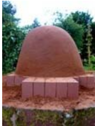
2) Build a sand dome
