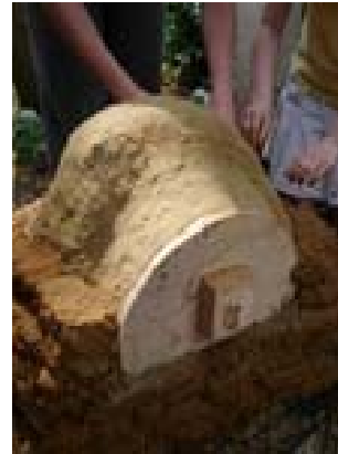
3) Cover with layers of cob
